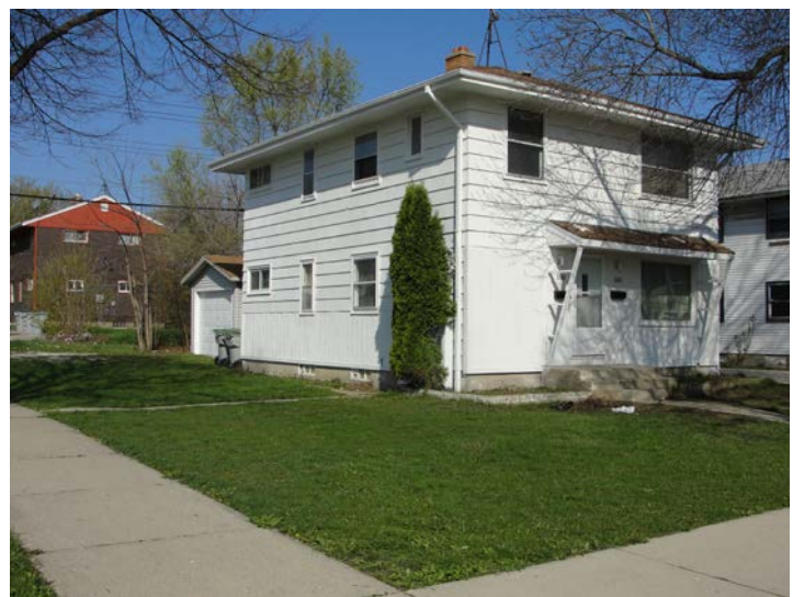
Same home after repair. (5641-5643 N. 61 st St.).
