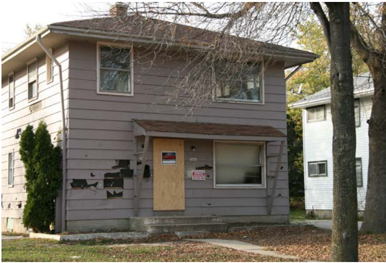
Abandoned housing in poor condition (5641-5643 N. 61 st St.).
